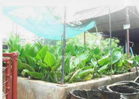
Constructed wetland for treatment of diethylene glycol contaminated wastewater by Burhead plant
